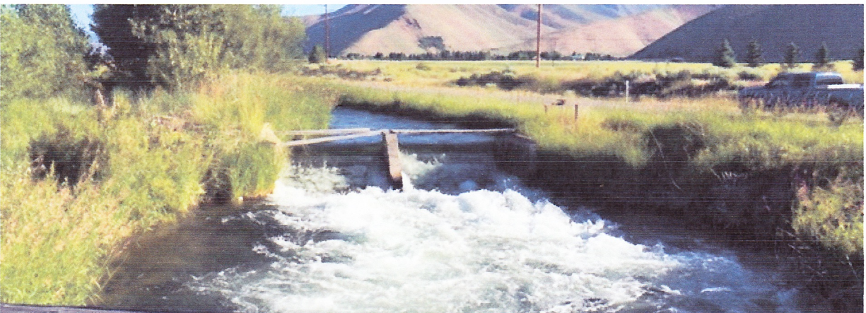
Center Lateral above Lab Lane
