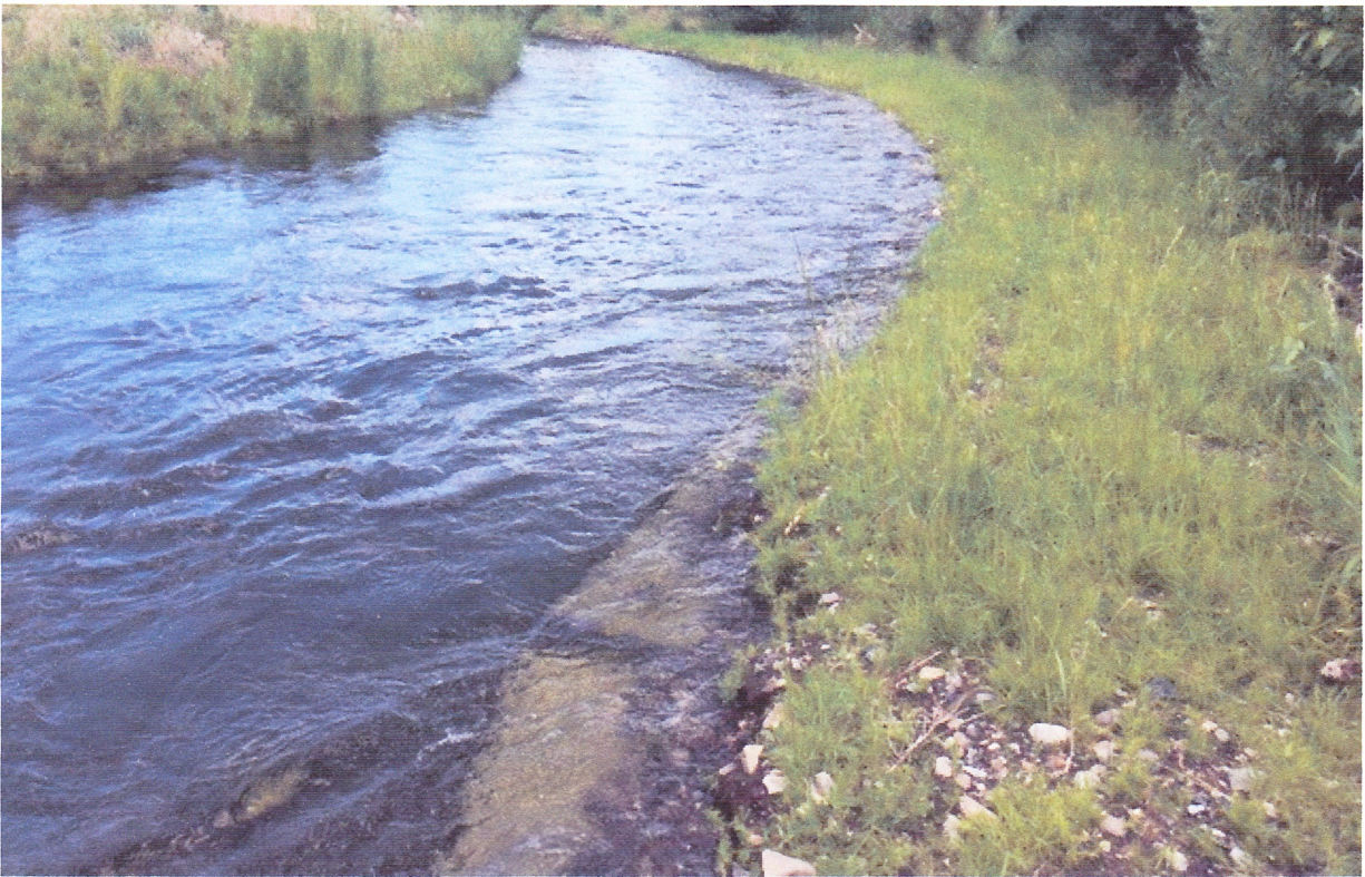
Our new wall just south of town
