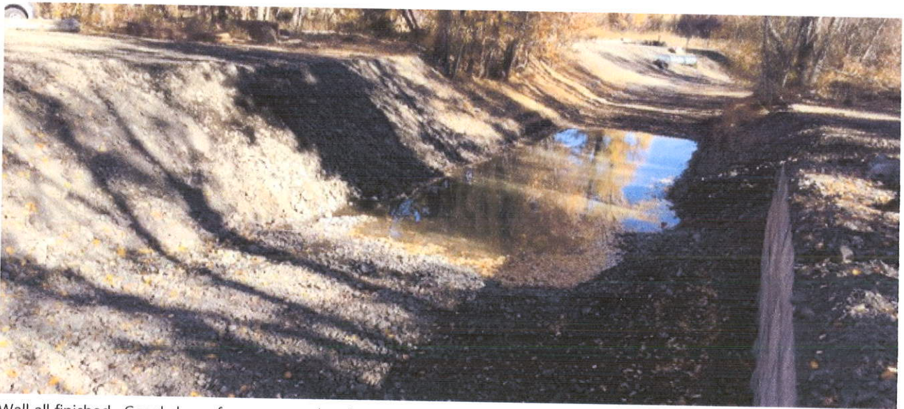
Wall all finished. Canal clear of excess gravel and equipment.
