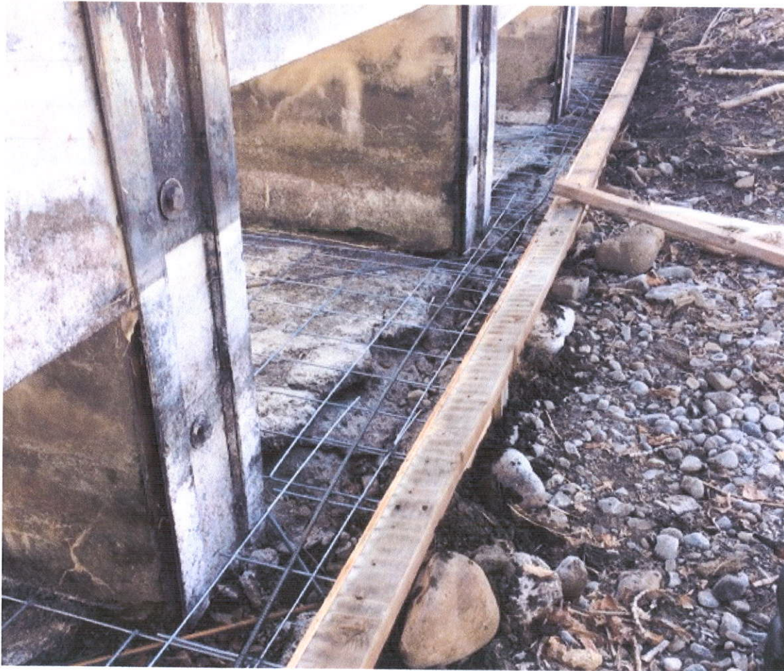
Chris directed us in setting up forms for a new floor.
