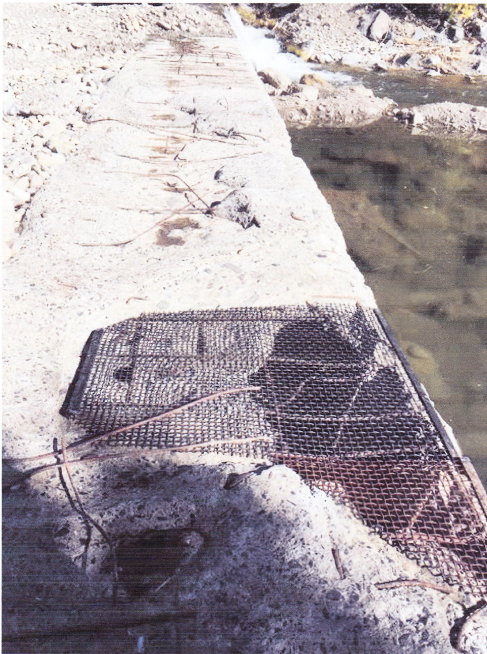
Cover up the holes. Note the exposed rebar and the fact that the structure is hollow
