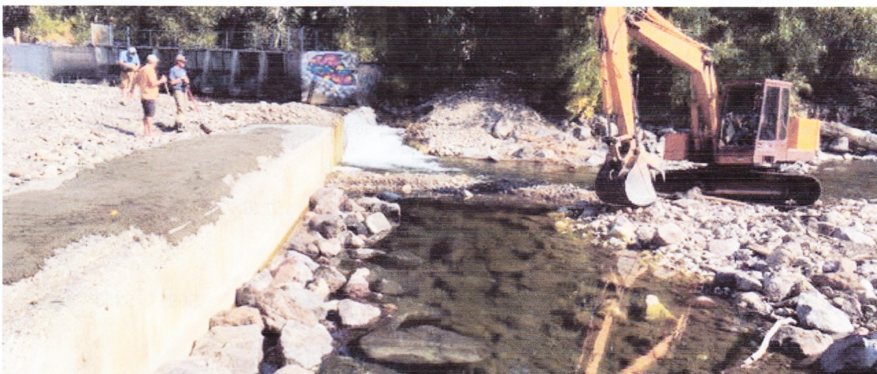
Replacing the old chunks of riprap back up against the lower side of the dam. This is also a very temporary "clean-up" simply done to buy us a little more time to come up with a long term repair.
