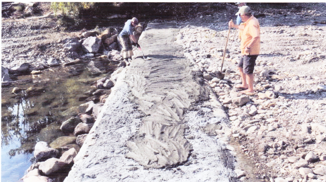
Rough patch of cement to cover the exposed rebar and holes. This will make it safer to leave as is while we develop a plan to address it more permanently.
