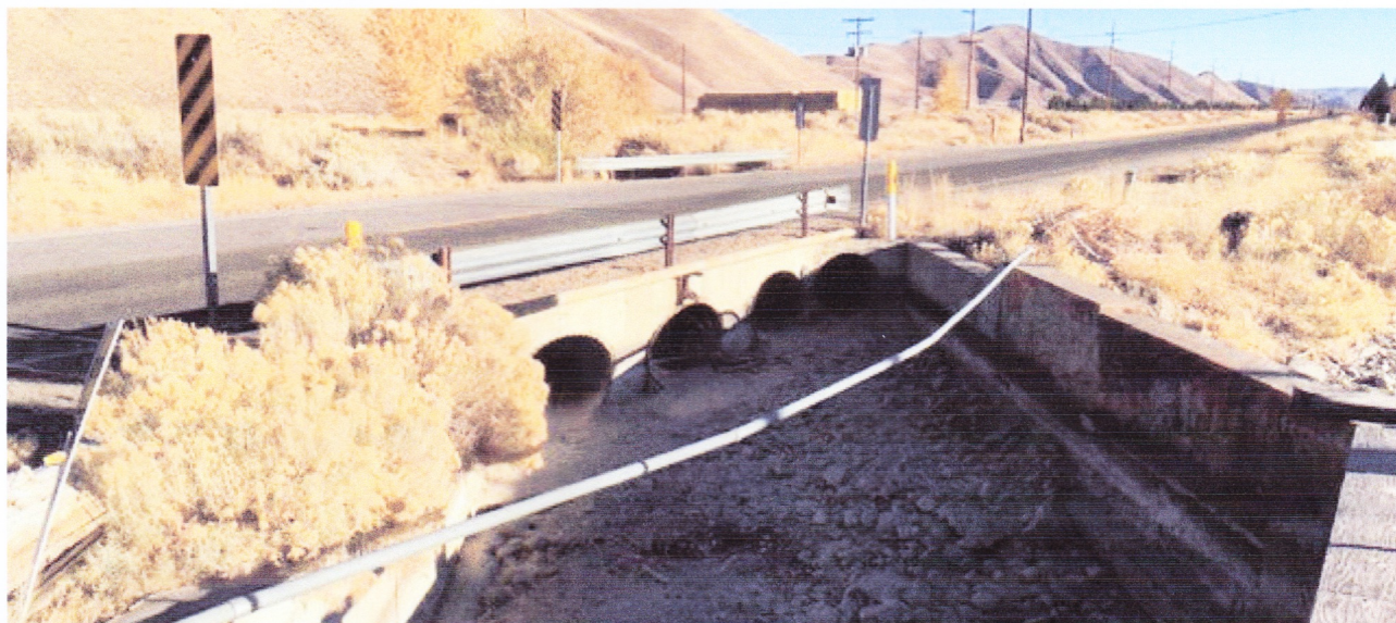
Intermountain Gas is placing their conduit, which is attached to the bridge, under the canal. The hanging conduit belongs to Century Link. I've asked Century Link to reroute theirs in order to hang it along the side of the bridge to neaten it all up and reduce risk.
